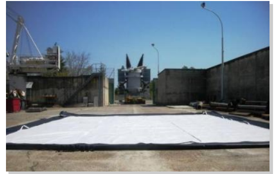
3 - Positioning the geo-textile sheet
