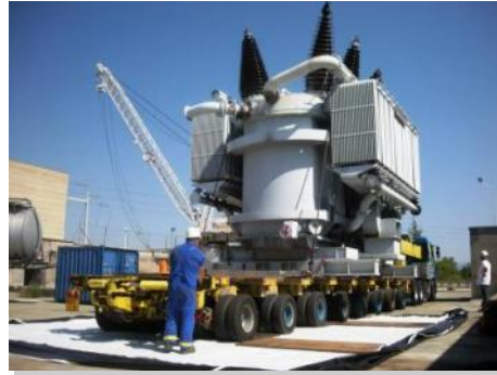
5 - Rolling the transformer into place
