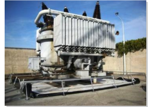
6 - Assembling the tank
