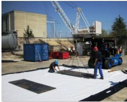
4 - Positioning load bearing plates
