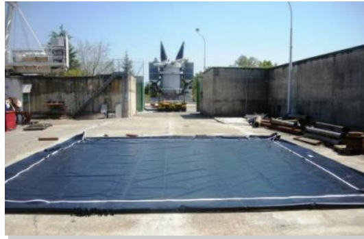
2 - Unrolling the tank
